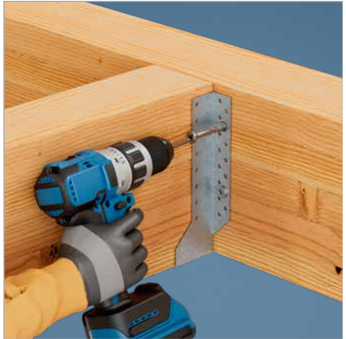
SSF screws fastening of BSNN joist hanger.
