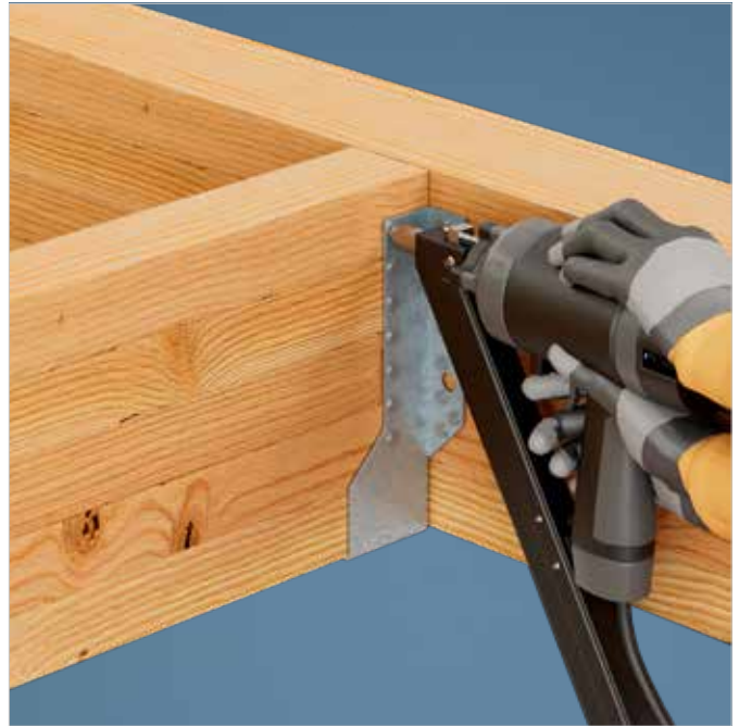
CNA connectors nails used to fasten joist hanger.
