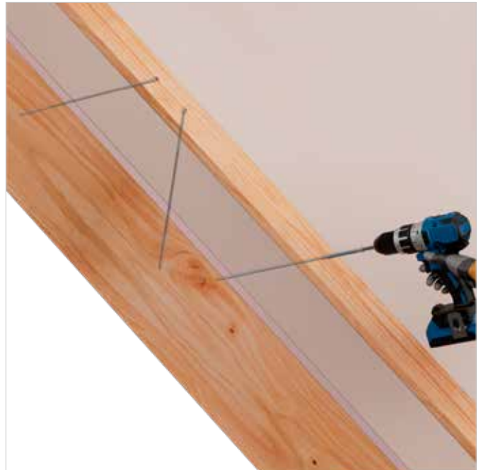
SWRS screws in rafter insulation application.
