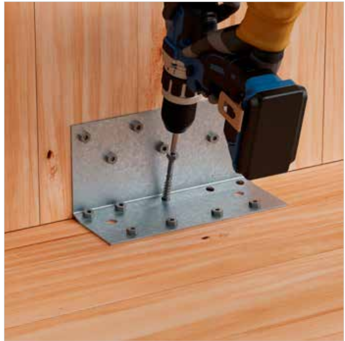
SSH screws fastening of AB255SSH angle bracket.
