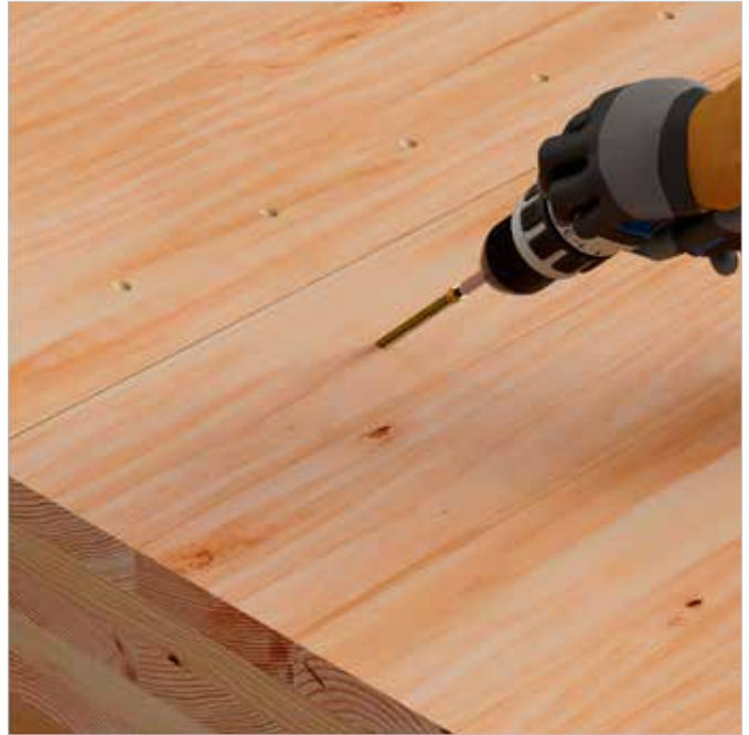
ESCRFTZ screws in installation of CLT butt-joint application.
